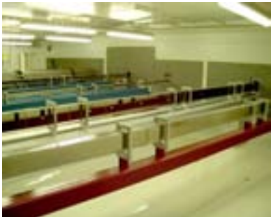
Figure 1.8: the completed casemate wall. The individual NG running through the casemate pass the wall towards the NG hall.
