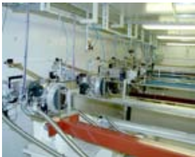
Figure 1.6: The tunnel wall, seen from the casemate side after completion. The vacuum tubes sticking out of the steel plates are connected with the high speed shutters. At their exit the vacuum tight NG follow, which are supported by the steel bars (first one is brown).
