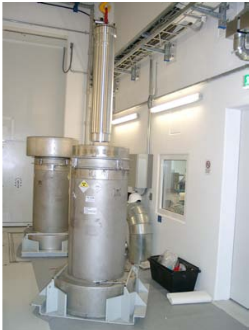
Figure 1.15: Pulling out of a fuel rod from a transportation container in the truck lock of FRM-II.
