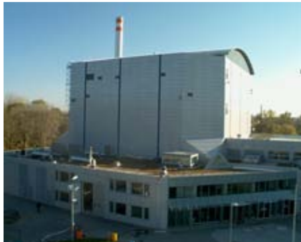
30.10.03 The FRM-II building in October 2003
