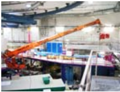
Figure 5.4: Mounting the blockhouse roof elements with a truck-mounted crane
