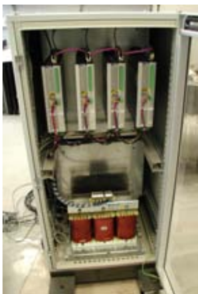
Figure 5.7: Control unit for the manipulators.
