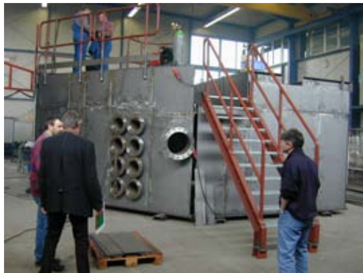
Figure 3.17: The instrument chamber during an inspection in March
