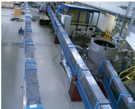
Figure 1.5: View of the NG NL 5, NL 6a and NL 6b in the NG hall. After having introduced the boron epoxy layers directly around the glass elements, the lead shield of originally 7cm thickness has been reinforced by several layers of lead plates, each 25 mm thick.
