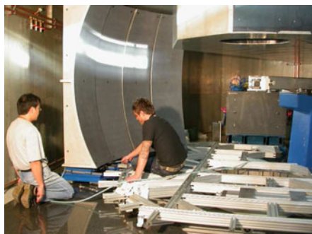
Figure 3.7: Installing the large-angle reflectors
