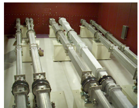
Figure 1.9: View of the NG in the tunnel area. The more bright colour of vacuum housing of NL 4a,b indicates the aluminium material.
