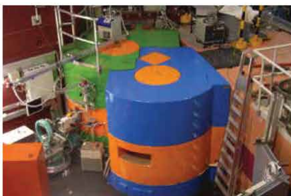
Figure 3: Biological shielding of POLI installed at beam tube SR9a.
