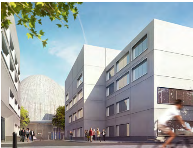
Figure 1: The axis between workshop and office building (left) and laboratory and office building (right) affords a view of the heritage-listed "Atomic Egg".
