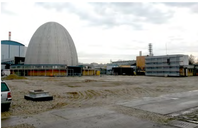
Figure 2: Cleared construction site for a new workshop, office and laboratory buildings.
