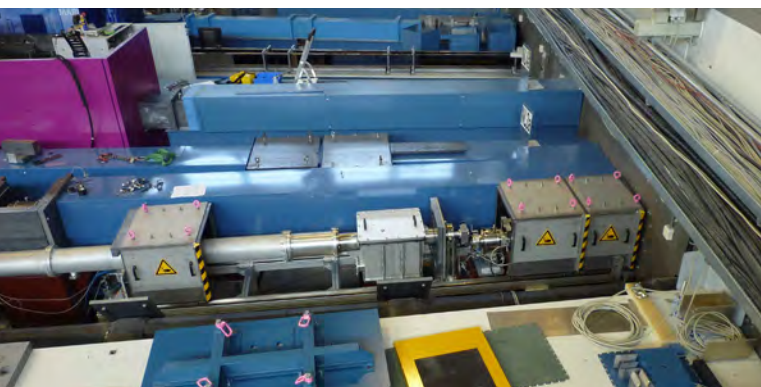
Fig. 1a: New mobile shielding installed at KWS-3.
